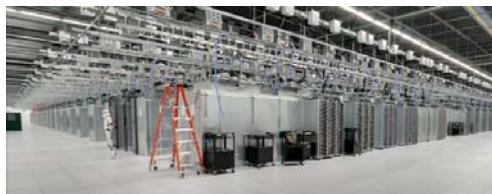
Google data center
